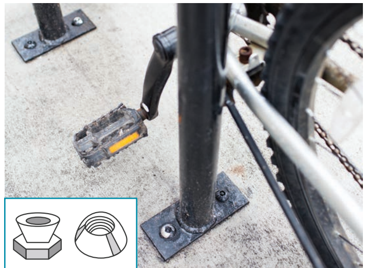
Flange (Surface) Mount and Tamper Resistant Nuts
